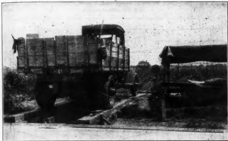
FIG. 2.—RUNWAY AND AUXILIARY TRUCK FOR APPLYING EQUIVALENT STATIC LOAD AT POINT OF IMPACT.
