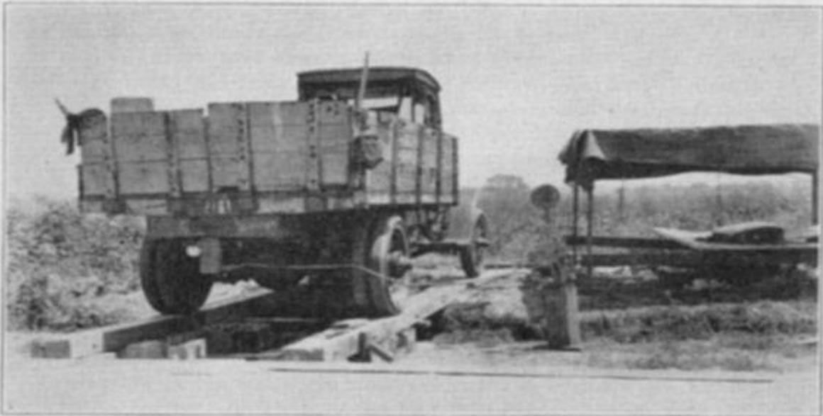
FIG. 2.—RUNWAY AND AUXILIARY TRUCK FOR APPLYING EQUIVALENT STATIC LOAD AT POINT OF IMPACT.
