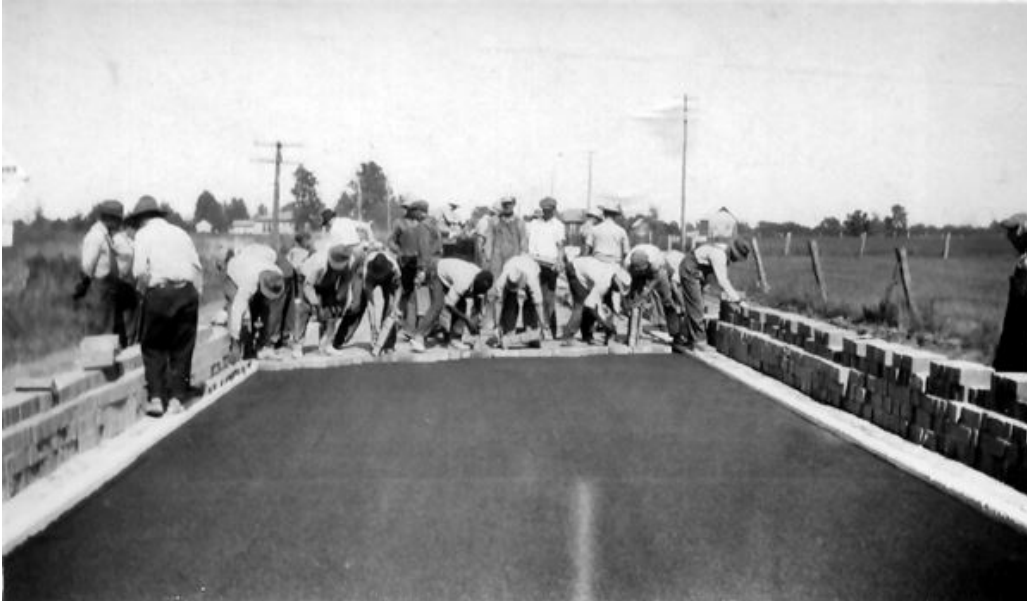
Road building crew laying bricks 1920s in Illinois. Credits
