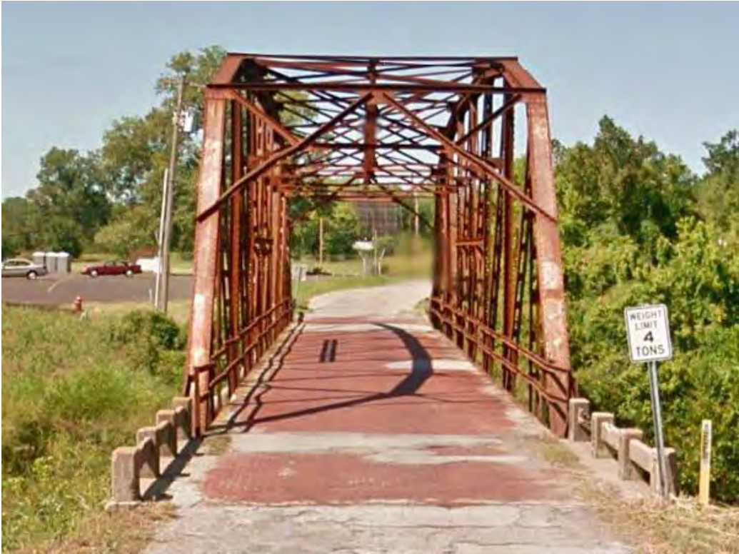
Rock Creek Bridge in Sapulpa (notice the "brick decking" or paving). Click image for St. View
