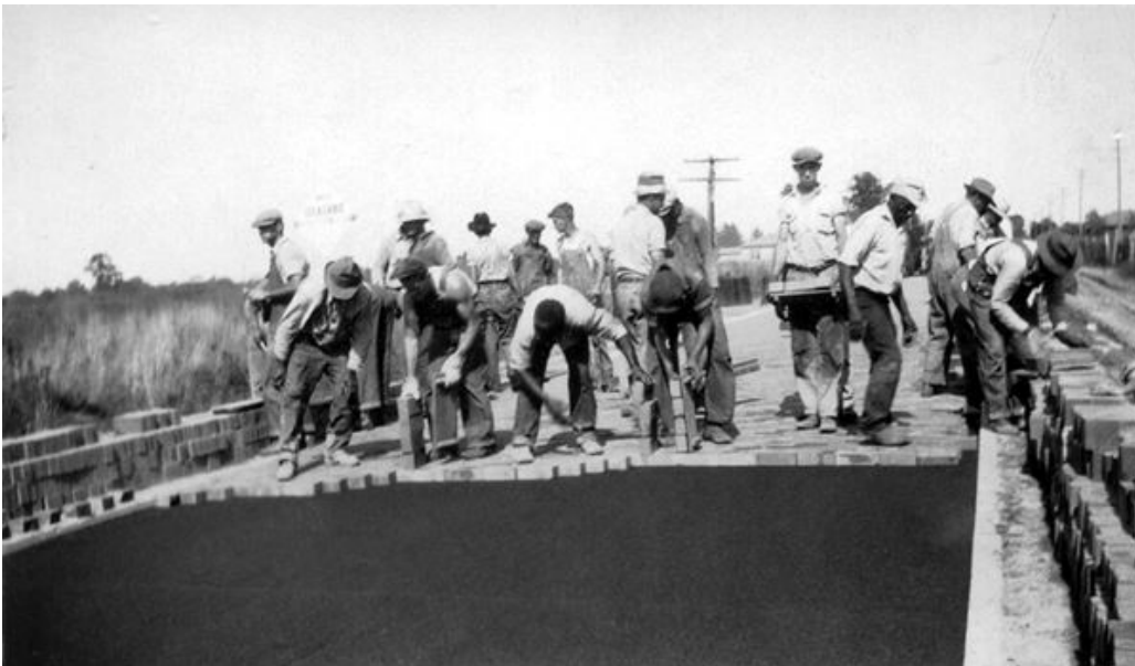
Men laying bricks 1920s. Illinois. Credits
