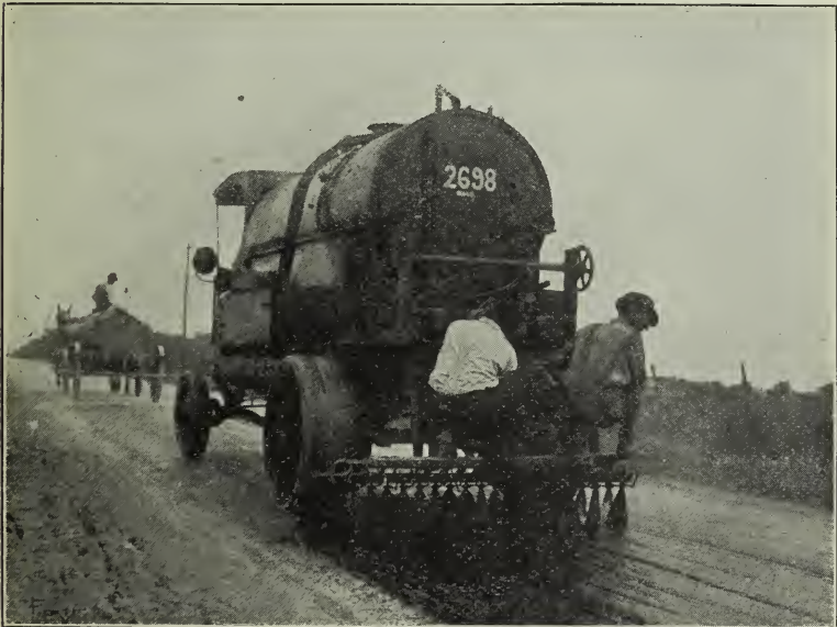
Fig. 20. Eight Hundred Gallon Auto Pressure Oil Distributor For Applying Cold Oil.
