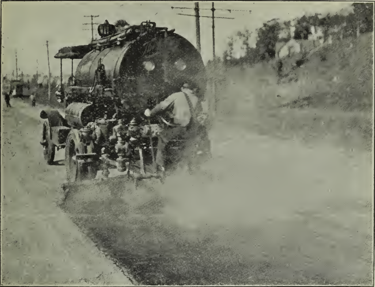
Fig. 19. One Thousand Gallon Auto Pressure Oil Distributor For Applying Hot or Cold Oil. Such Equipment Has Been Used in Distributing Oil 25 Miles From the Supply.
