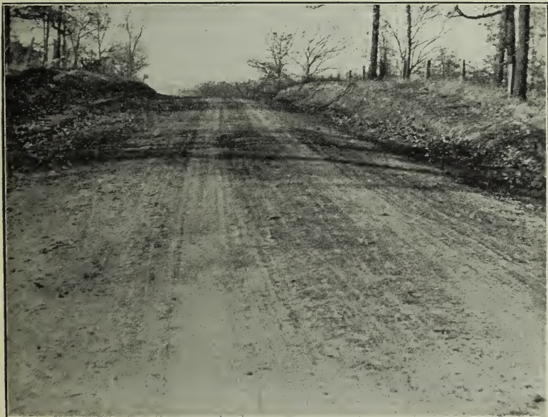
Fig. 4. Oiled Earth Road in Spring of the Second Year. Surface is Kept Smooth by Means of Light Drag. The Continued Use of a Light Drag is of Great Benefit.
