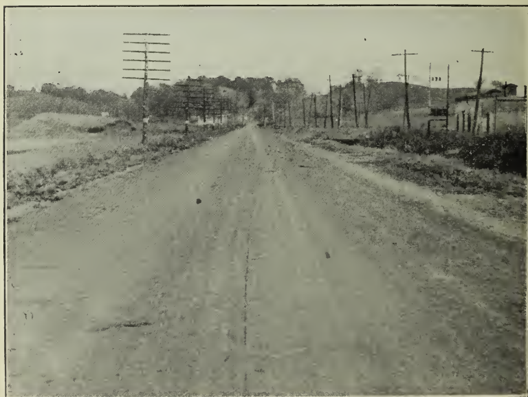
Fig. 26. Macadam Road Maintained Under Heavy Traffic by Means of Annual Treatments of a Bituminous Material and Coarse Sand.
