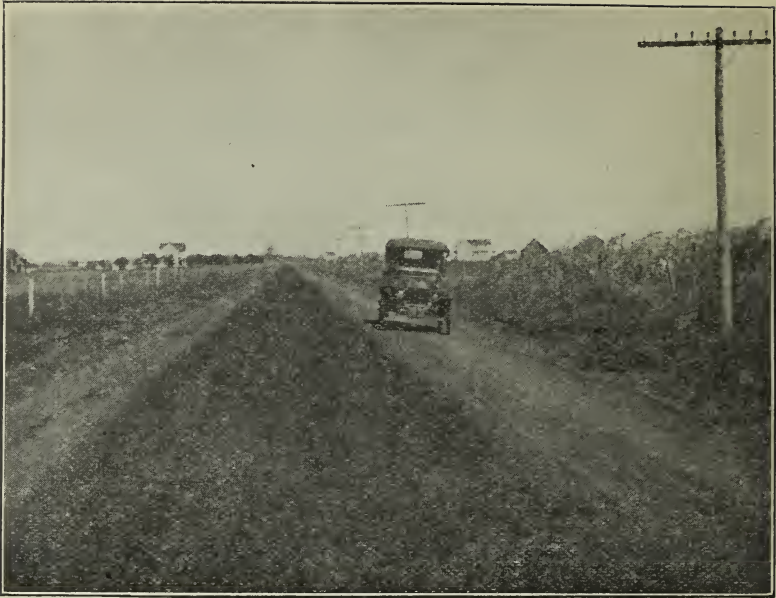
Fig. 1. Oiled Earth Road 15 Feet Wide After First Treatment of Three-eighths Gallon Per Square Yard. Note the Road Was Well Graded and Shaped Before Oil Was Applied. Such Work Insures The Best Results.
