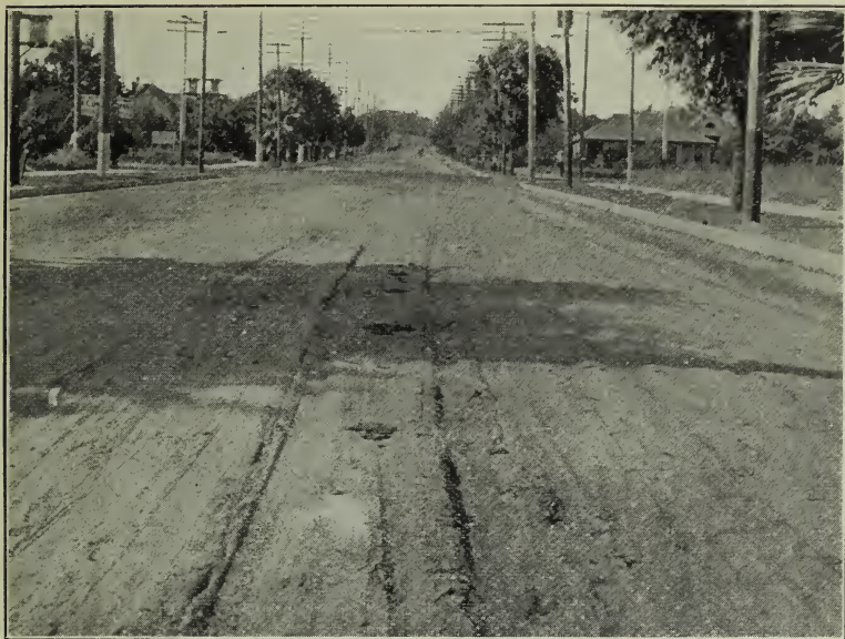
Fig. 23. Oiled Sand Road in California. Surface Not Entirely Satisfactory on Account of the Greasy Oil Used.
