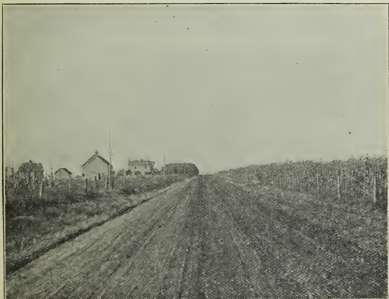
Fig. 10. Oiled Earth Road After Two Weeks of Summer Rains. Surface in Excellent Condition. Note Uniform Grade and Crown of Road.
