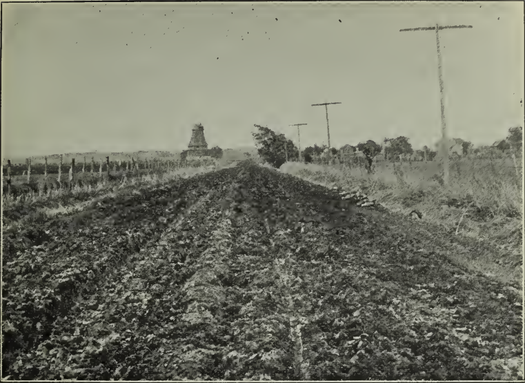
Fig. 7. A Well Graded Earth Road But Badly Cut Up at Time Picture Was Taken. It Should be Carefully Dragged and Compacted Under Heavy Roller Before Oiling. A Uniformly Compacted Surface Will Show the Best Results After Oiling.
