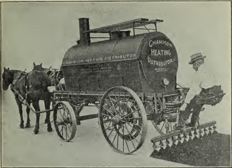
Fig. 13. Pressure Distributor For Applying Hot Oil. Heat Supplied by Oil Burners.
