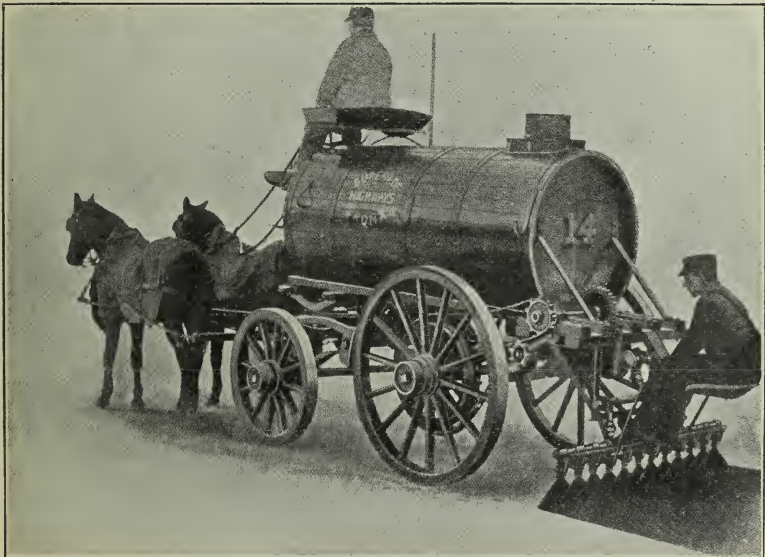
Fig. 14. Pressure Distributor For Applying Cold Oil. The Spraying Attachment Can be Attached to an Ordinary Tank Wagon as Shown in the Cut.
