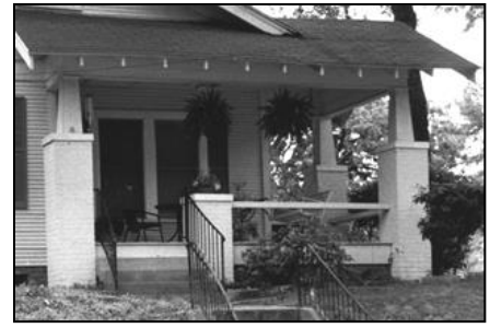
Tapered box supports on brick piers
