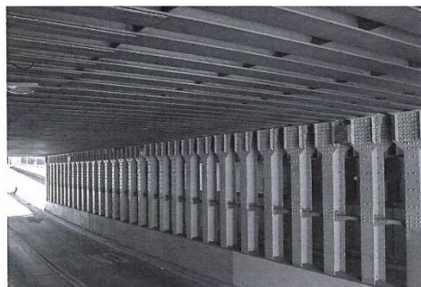
Left: The new raised tracks of the underpass take shape in 1937. (Hanna & Hanna photo, 1937, Albuquerque Museum, gift of Albuquerque National Bank) Right: Three rows of steel columns support the bridge over the underpass. Columns rest on piles driven 30 to 40 feet into the underlying sand. (Roger Zimmerman photo)
