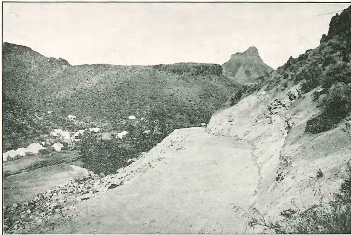
MOHAVE COUNTY Kingman-Oatman Highway, Showing Roadway After Blasting Away Rock
