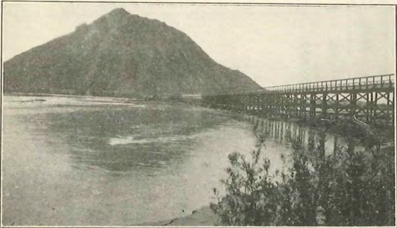
ANTELOPE BRIDGE—REBUILT WITH 55-FOOT PILES
