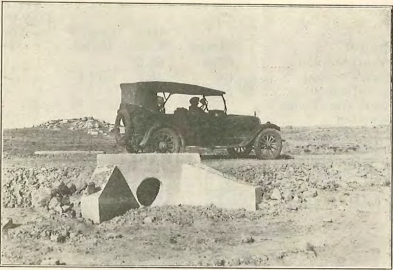
STANDARD CULVERT—HOLBROOK-ST. JOHNS HIGHWAY
