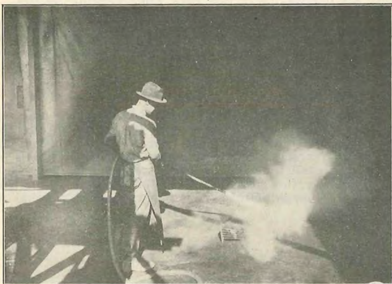
HOT WATER JET—FOR CLEANING MOTOR PARTS.
