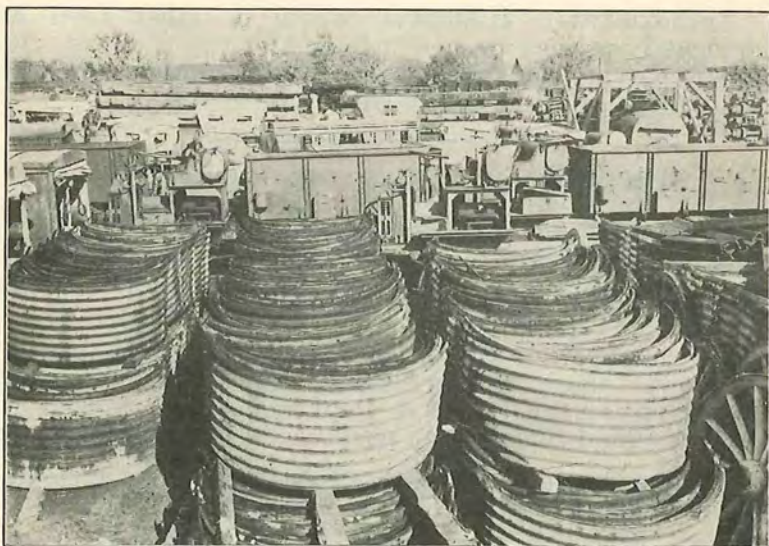
ONE MAN ARMY SHELTERS—USED FOR CULVERTS.
