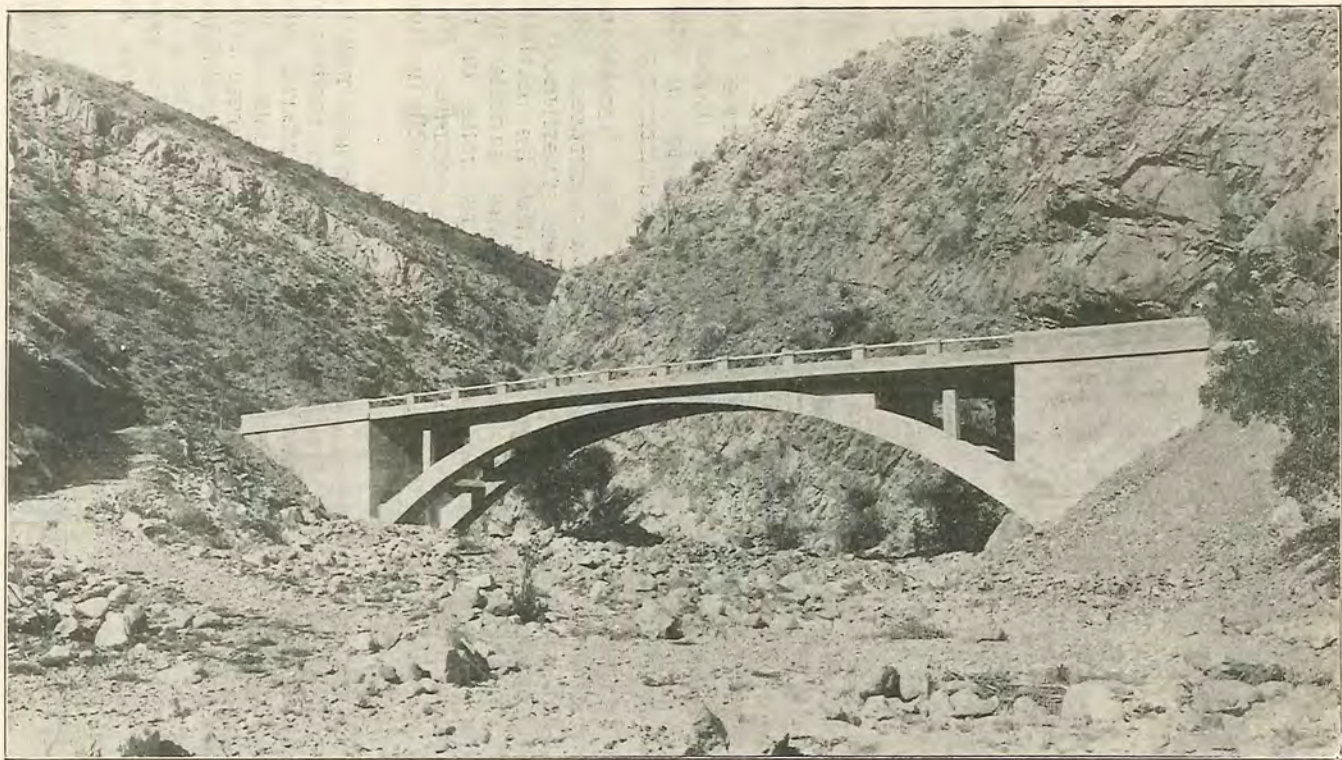
UPPER QUEEN CREEK—SUPERIOR-MIAMI HIGHWAY. TWO RIBBER RE-INFORCED CONCRETE ARCH.
