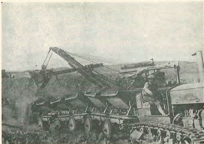
SURFACING PHOENIX-YUMA HIGHWAY FROM GRAVEL PIT
