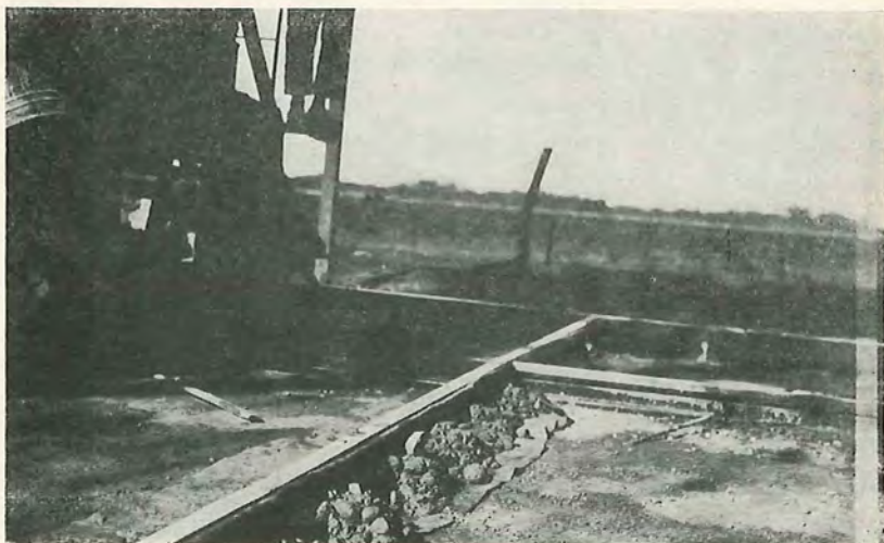
CONSTRUCTION OF PAVEMENT JOINT
