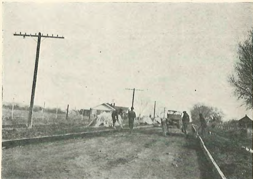
PREPARING SUBGRADE FOR PAVEMENT
