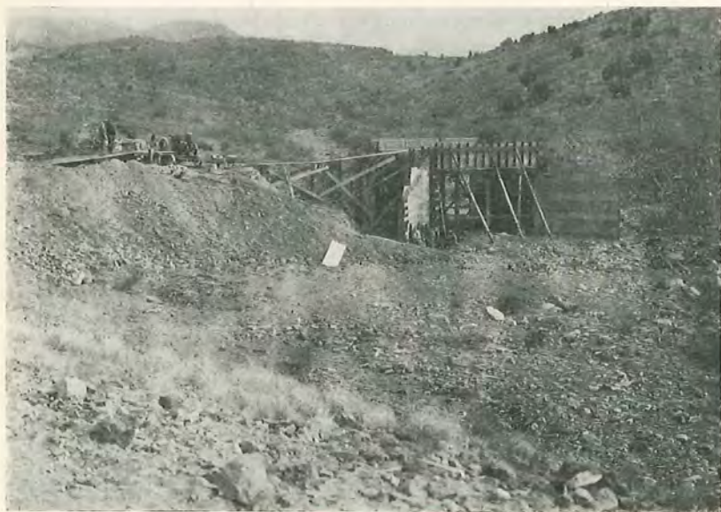
CONSTRUCTING A 20-FOOT SLAB BRIDGE
