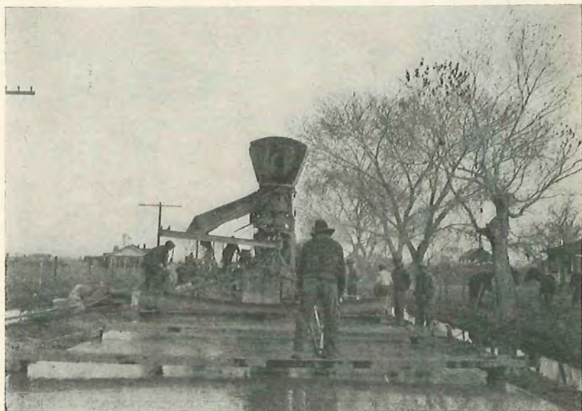
FINISHING CONCRETE PAVEMENT
