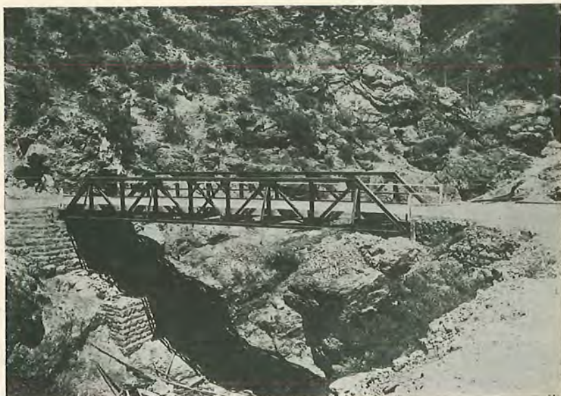
73-FOOT LOW TRUSS OVER FISH CREEK
