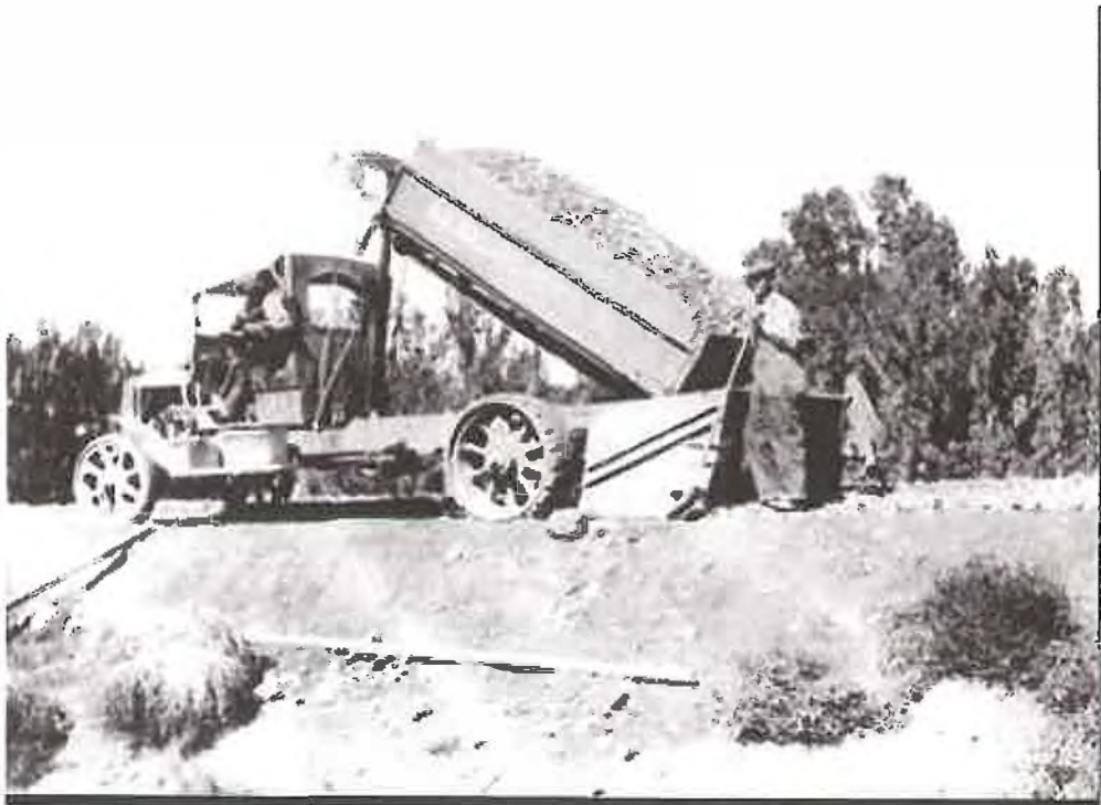
Placing Base on Route 66, 1926
